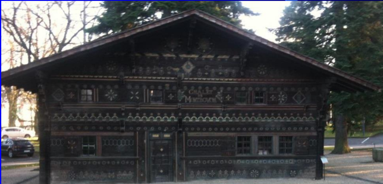
Swiss chalet presently located below the flags entrance
